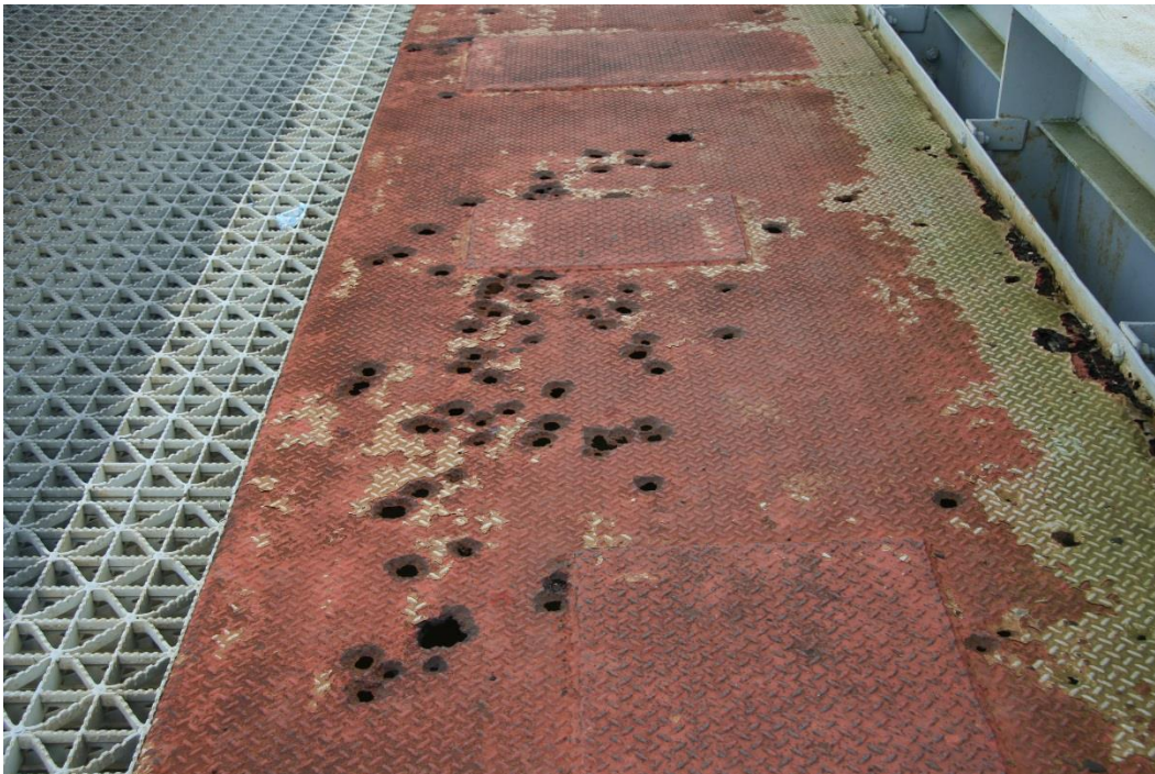
Condition Photo 15: Metal plate walkway condition, south walkway, west end.
