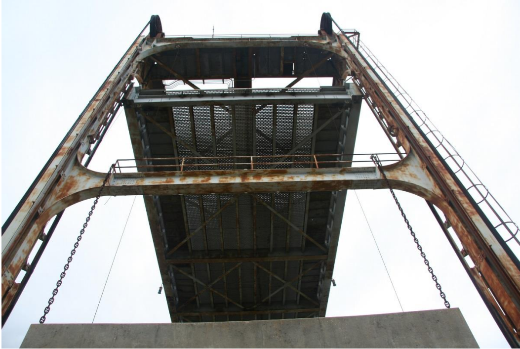
Condition Photo 6: East lift tower with bridge open.
