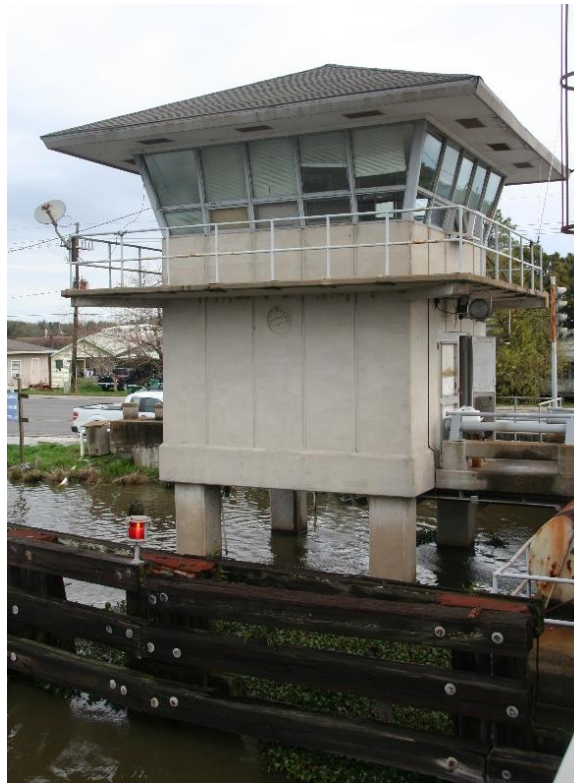
Condition Photo 17: Bridge operator's house, west side, looking east.
