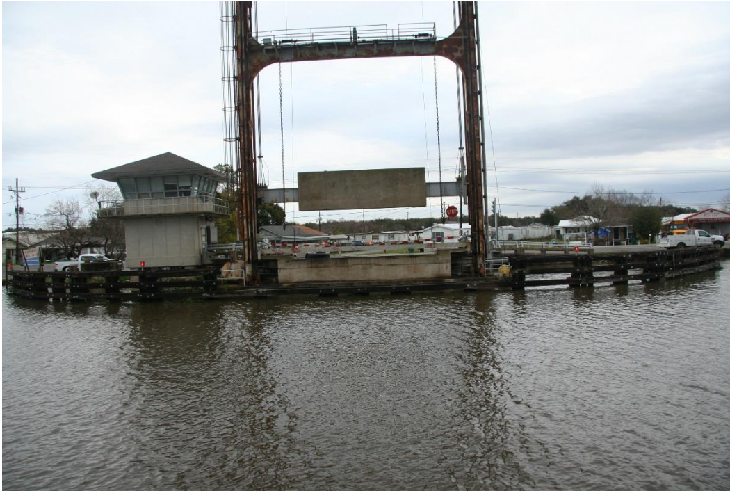
Condition Photo 12: East lift tower and timber fender system, looking east.
