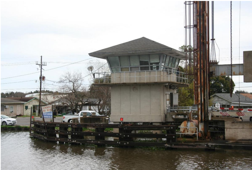
Condition Photo 11: Operator's house and northwest tower and timber fender system.
