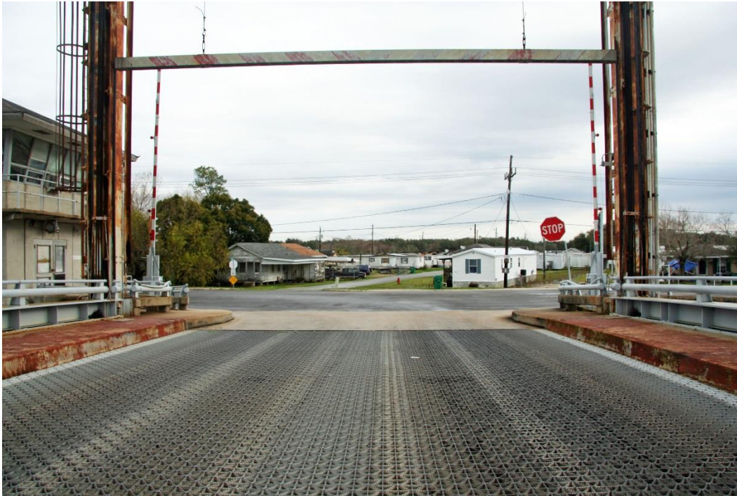
Condition Photo 2: Looking east from center of bridge at LA 308 intersection on east side of bridge.
