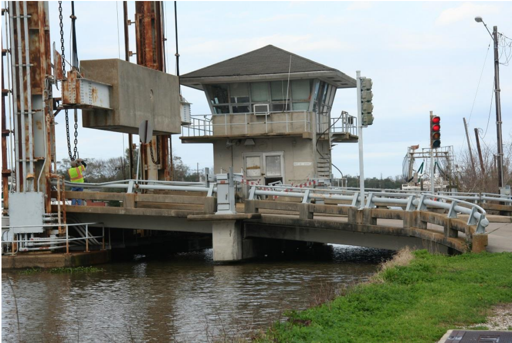
Condition Photo 4: Bridge operator's house and east approach spans at LA 308.
