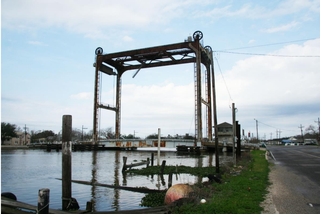
Character-defining Feature Photo 1: Design and construction of a vertical lift span with central drive machinery. The operating machinery, located at the center of a platform, drives the four sheaves on each corner of the lift towers. Note location of original operator's house on northeast quadrant of bridge.
