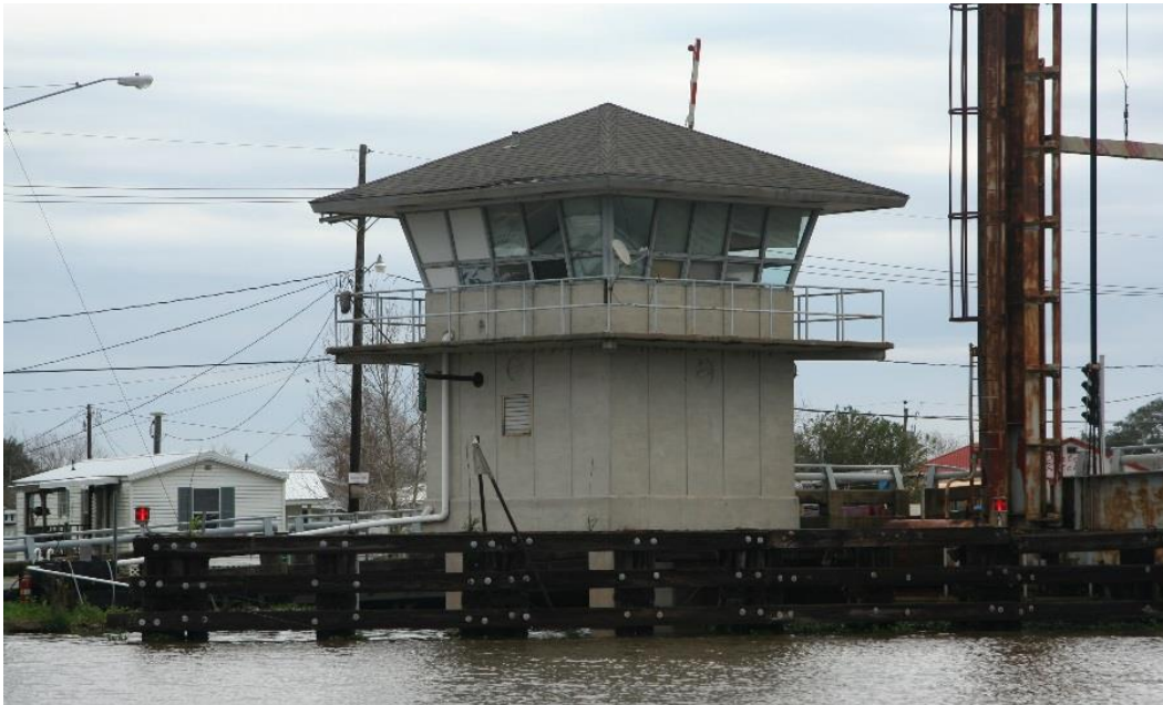
Historic Fabric Photo 1: Original two-story concrete operator's house. Details visible in this photo include cantilevered windows, vertically scribed concrete, brown pelican emblem, and balcony with metal railing.
